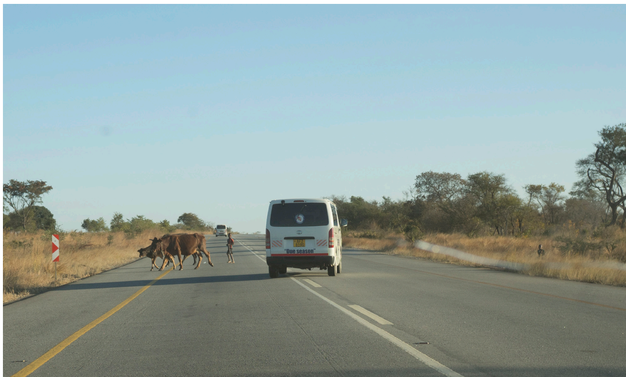
Figure 3: Harare to Beitbridge Road prior to and after Reconstruction
